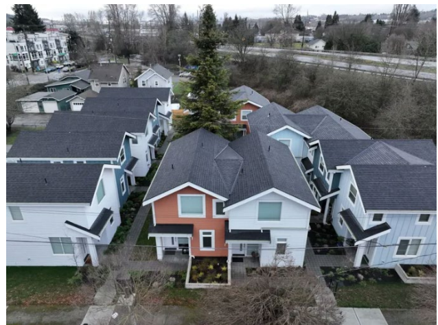
Figure 2 Habitat for Humanity Project. South Park, Seattle.
